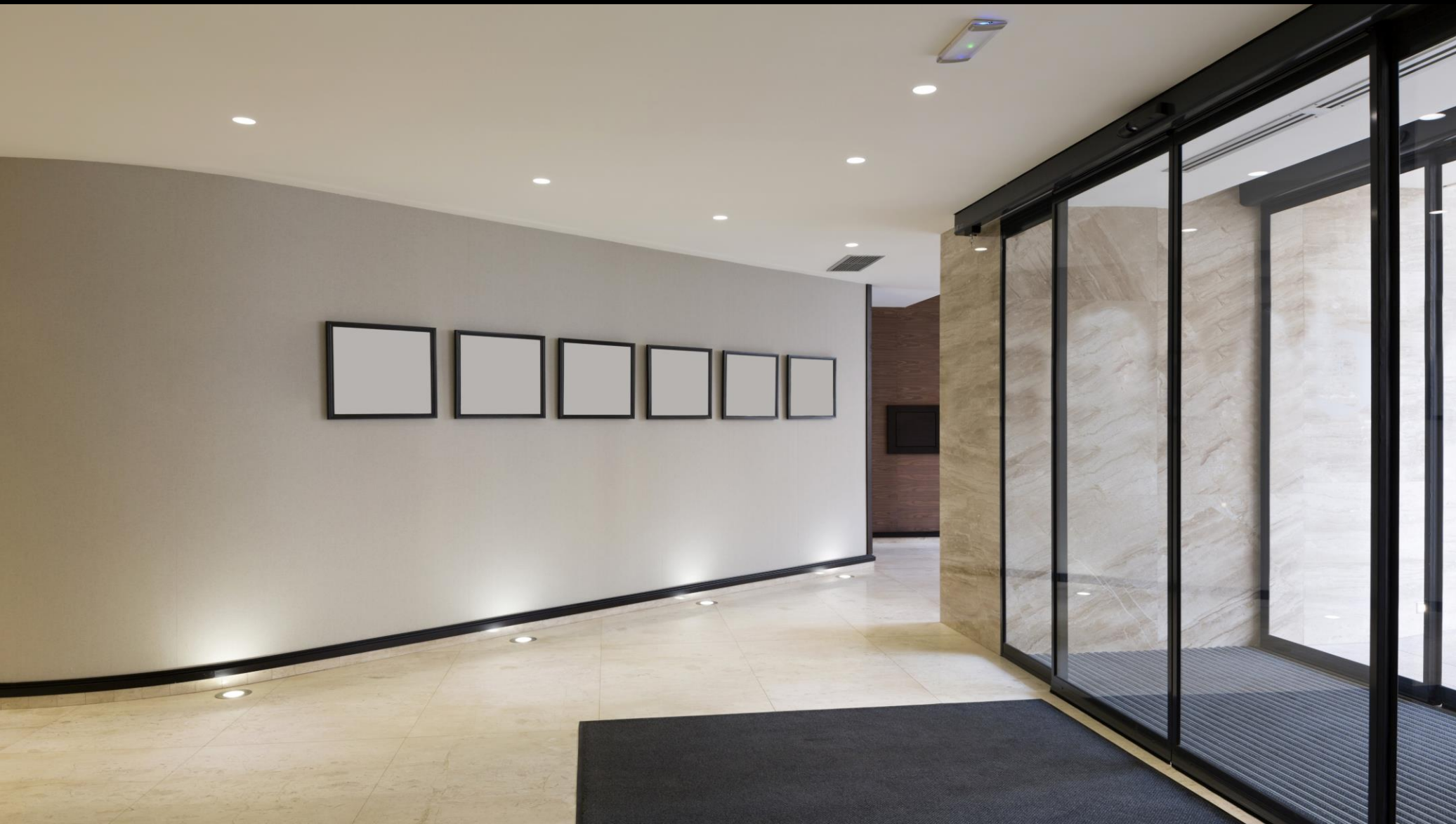
Small commercial downlights
